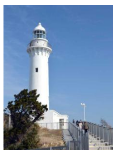
The lighthouse after the road has been repair
