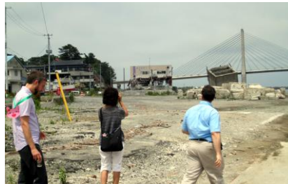
A visit to Port Haragama to inspect the tsunami hit areas.
